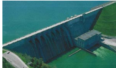
This dam is an example of a typical Tennessee Valley Authority hydroelectric/ flood control design. Next to some larger dams, TVA would construct a large coal-fired power plant. Such a combination adds additional modeling opportunities with a reason for large coal train based unloading facility like the Norris dam and Bull Run Fossil Plant. Watt Bar Dam includes locks for barge traffic and a Nuclear power Plant. The Watts Bar location was also considered as a site for an additional fossil plant.
