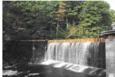
Kennebunk Light and Power represents low head hydroelectric generation in Maine. It was founded in the 1880's. Water wheels were used in many of these plants. If you want an older dam an over shot or under shot grain mill may be what your model railroad requires. Watt Bar Dam includes locks for barge traffic and a Nuclear power Plant. The Watts Bar location was also considered as a site for an additional fossil plant.
