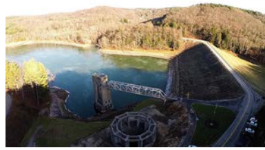
hydroelectric project around 2010. Photos of the cave like outlet are available on the Pleasant Hill website.
